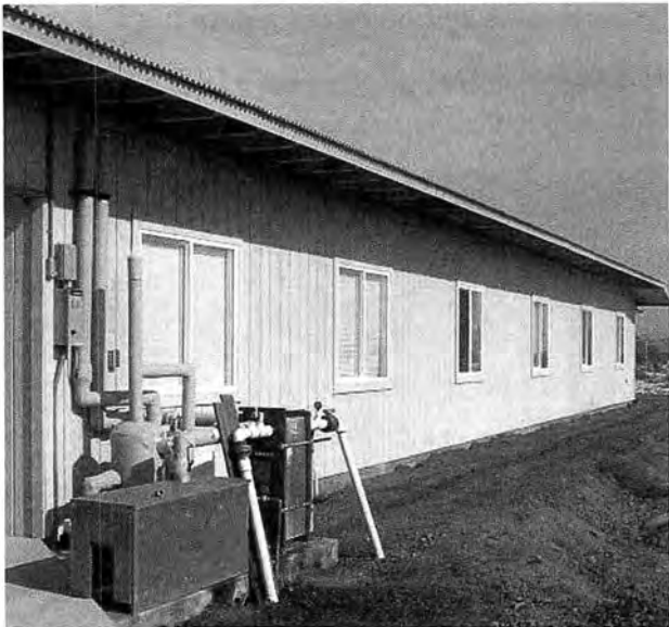
Fig. 4. A typical seawater A/C heat exchanger at a NELHA tenant facility
