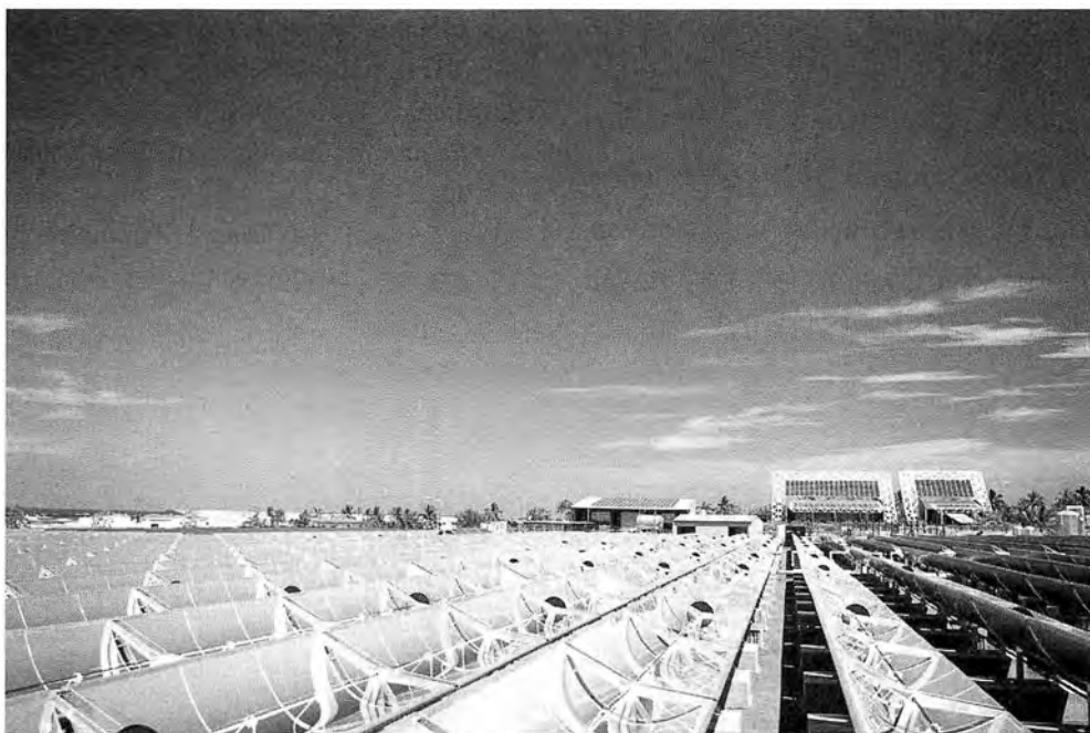
Fig. 3. 1008 solar thermal collectors are tracking the sun where the heat is used for a solar assisted OTEC system using an organic rankine cycle and NELHA's cold deep ocean water.
